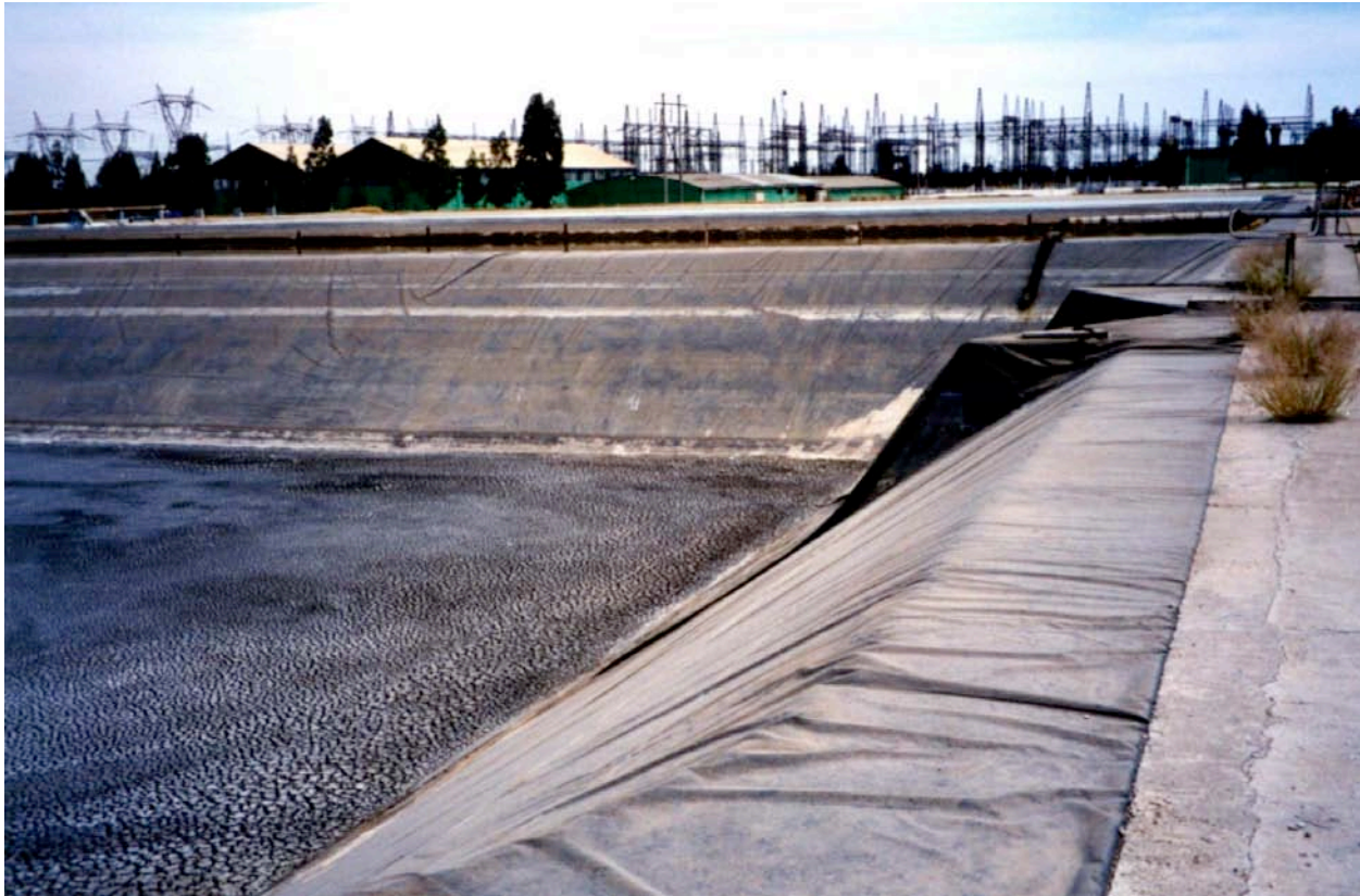
Figure 4 Geomembrane Perimeter Anchoring System and Outlet Structure
