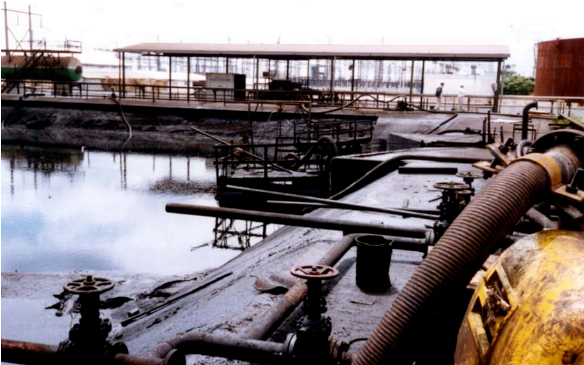
Figure 2 Impoundment prior to Lining
